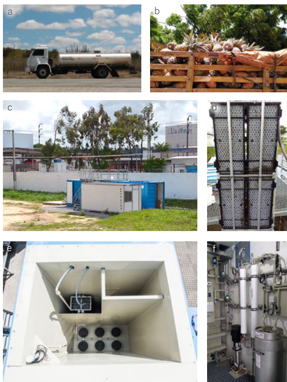
Figure 2: Impressions about the project BRAMAR and the MBR pilot plant installed by EnviroChemie GmbH in João Pessoa (Paraíba) to treat an industrial effluent coming from a fruit juice producing company.
