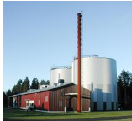
The biological wastewater treatment plant at Norrmejerier in Sweden
