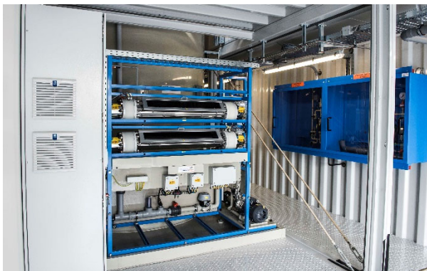
Removal of active pharmaceutical ingredients (API) using UV and hydrogen peroxide
