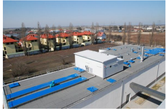
A compact plant solution – all treatment unit in one building
