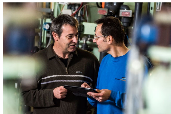
Image: An on-site contact for chemicals, sludge and spare parts reduces the invoicing and supplier negotiation workload
