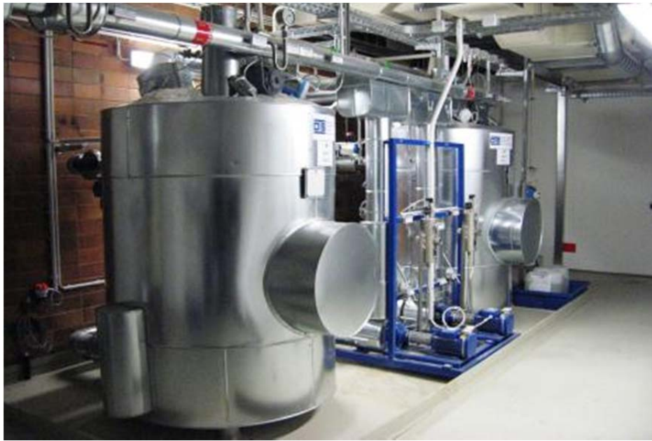
Figure 13. Batch thermal inactivation plant at Dessau-Tornau GmbH in Dessau (Germany). [Source: EnviroChemie GmbH]
