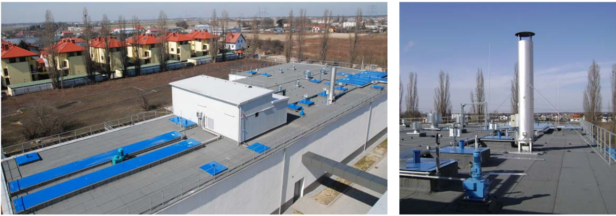
Figure 10. Overview of the WWTP implemented for Bioton S.A. (including detail of biogas flare). [Source: EnviroChemie GmbH]
